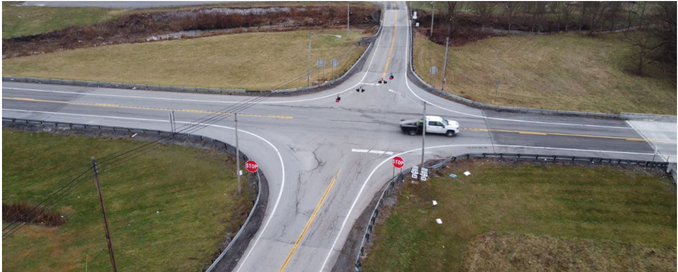
Figure 10: Flashing Beacon at KY 78 Intersection
